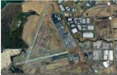
Figure 7: Land Availability is a major consideration. The area near the airport and Tank Farm Road appears the most promising.
